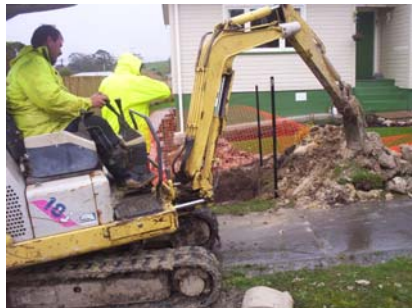
2006 New Potable Water Installation
